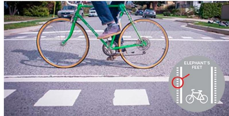
Elephants' Feet markings are used to indicate where cyclists are permitted to cross an intersection without dismounting and walking. Markings are painted white squares, placed either outside the white lines of a pedestrian crosswalk, or on one side of the pedestrian crossing.
