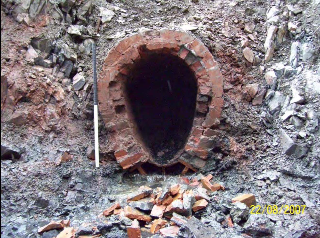
The earliest sewers all emptied directly into the harbour. But, after the City of St. John's was incorporated in 1888, one of the first orders of business was to construct an interceptor (or collector) sewer installed under Water Street. It was built using two methods: either an egg-shaped, double-walled brick pipe, or by tunneling through solid rock.
