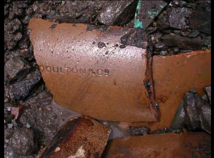
In the downtown core, the channels for the brooks were more elaborate, such as this stone-built sewer with a ceramic base, which carried Bells Chute into Ayres Cove from about 1860 – datable by the ceramic base, manufactured by Doulton & Co. of Lambeth, South London – who moved on from the manufacture of sewer pipes to become fine china makers Royal Doulton.
