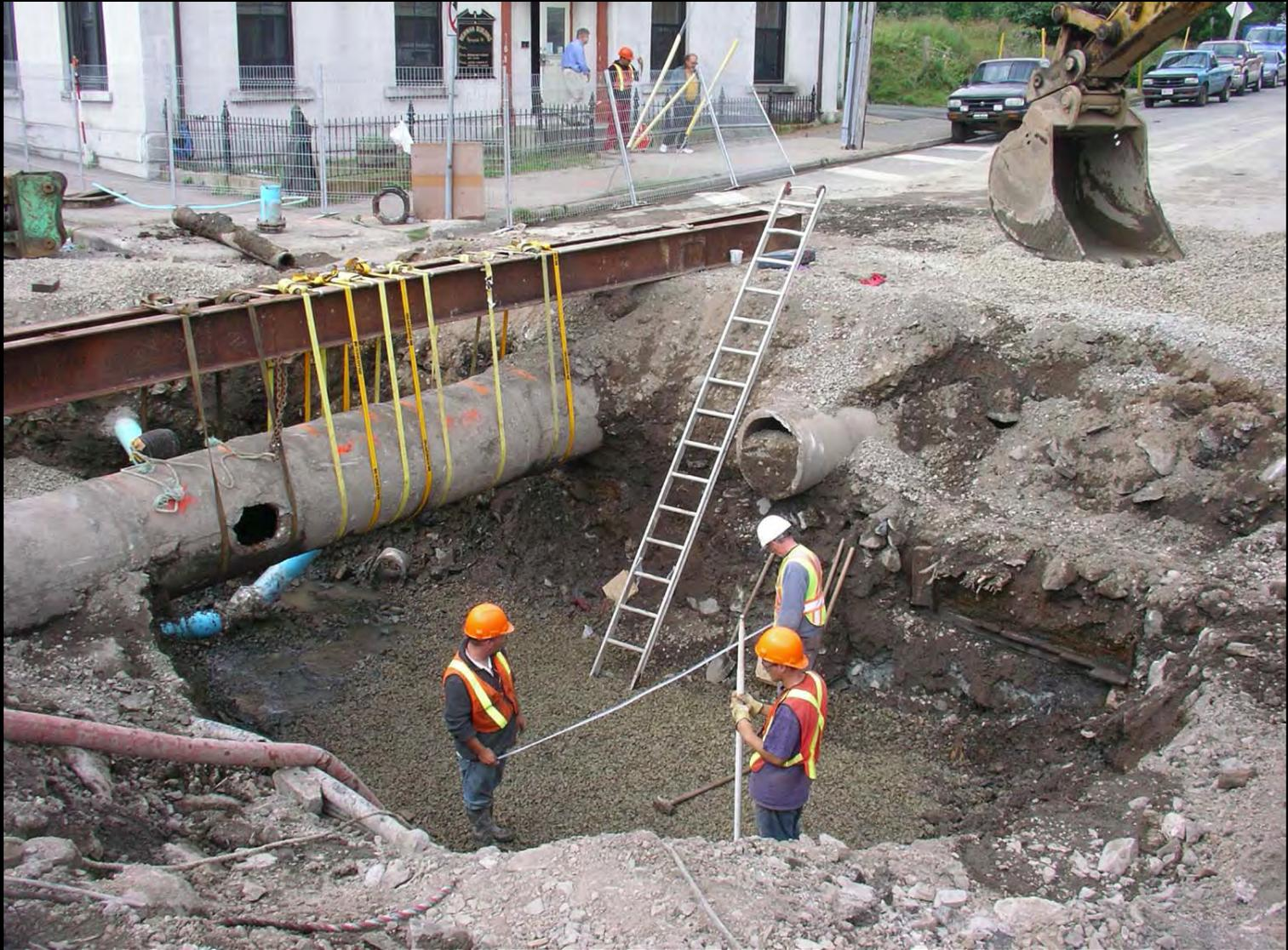
Phase 1 sewer pipe installation adjacent to the Newman building at the junction of Springdale Street and Water Street. Note the wooden “sluice” drain bottom right.
