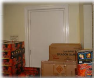
FIGURE 2a. Improper manner to store fireworks. There is no sign indicating fireworks storage, an exit is not identified and the exit is obstructed.
