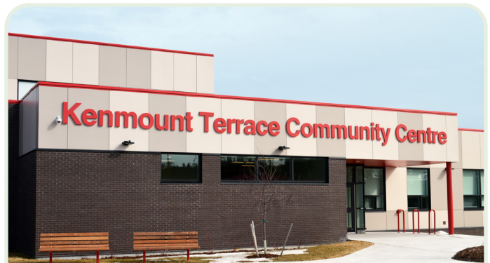
Kenmount Terrace Community Centre Exterior
