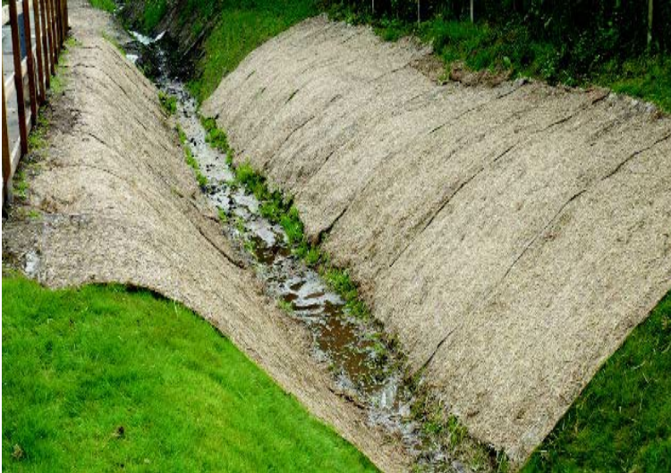
Figure 10-4 - Erosion Control Blanket
