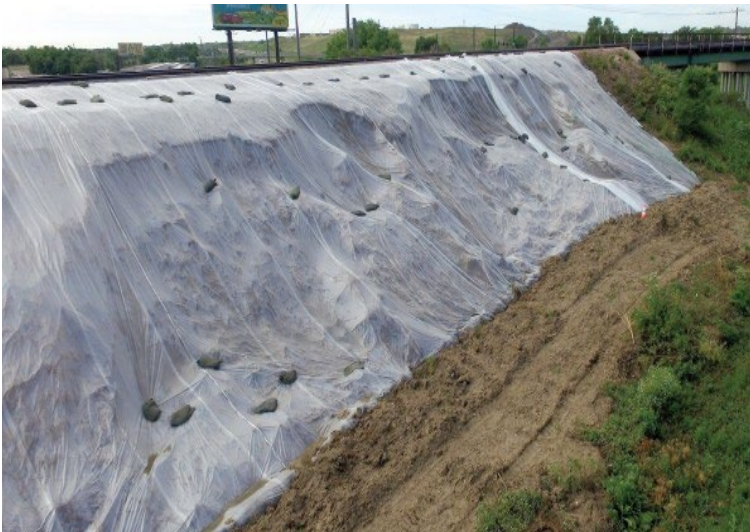
Figure 10-5 - Plastic Sheet covering
