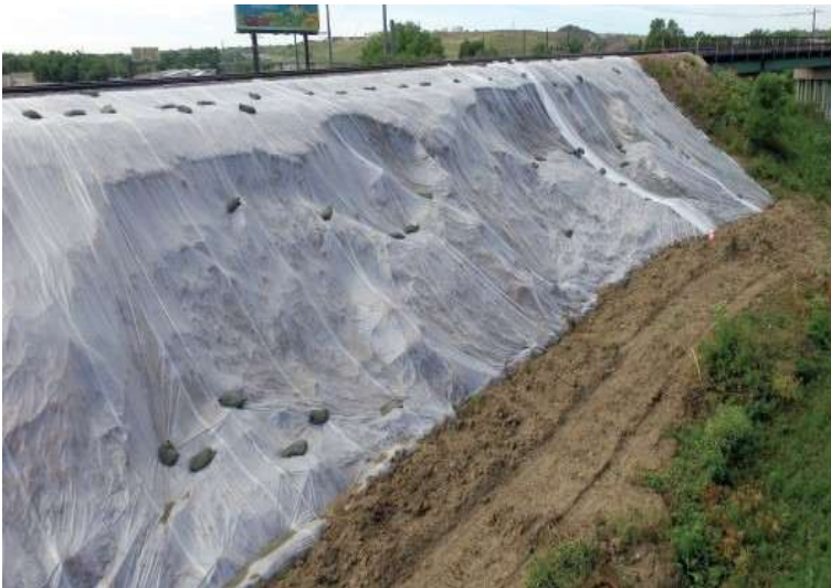
Figure 10-5 - Plastic Sheet Covering
